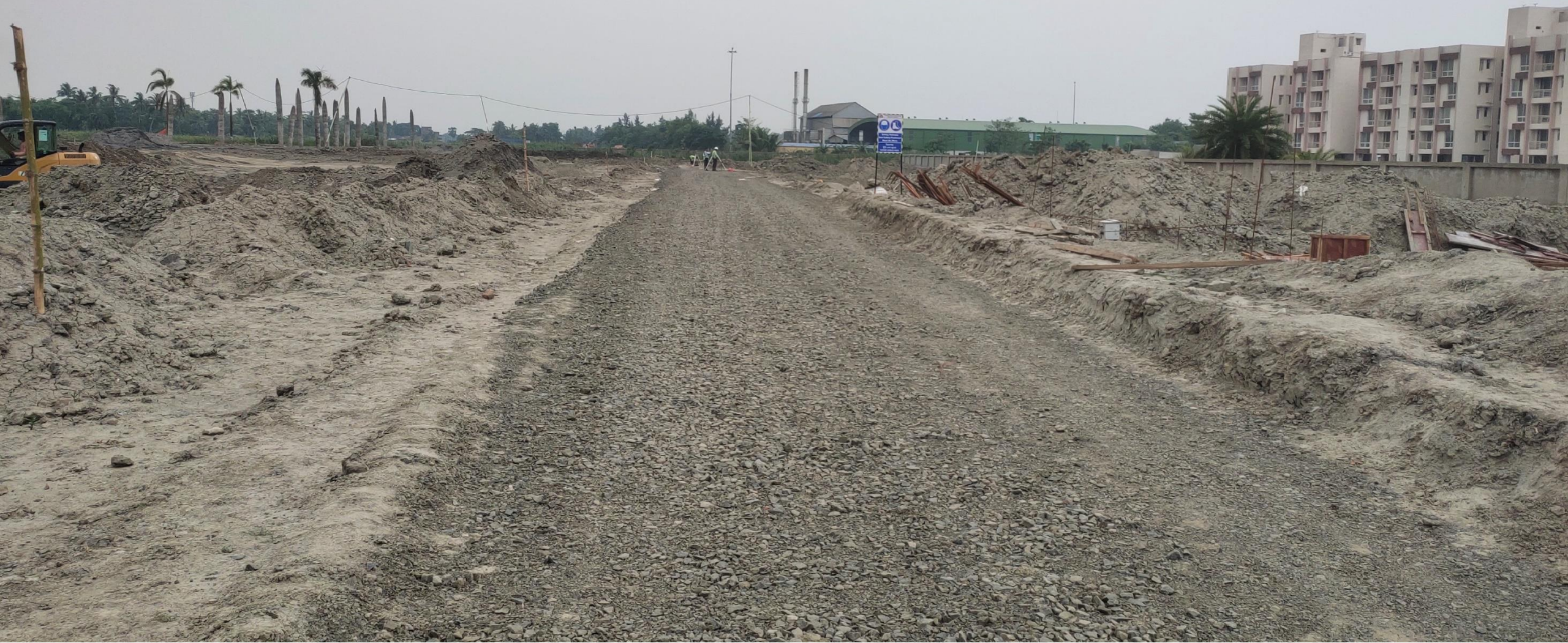
PROGRESS PHOTOGRAPHS: INTERNAL ROAD WORKS IN PROGRESS
