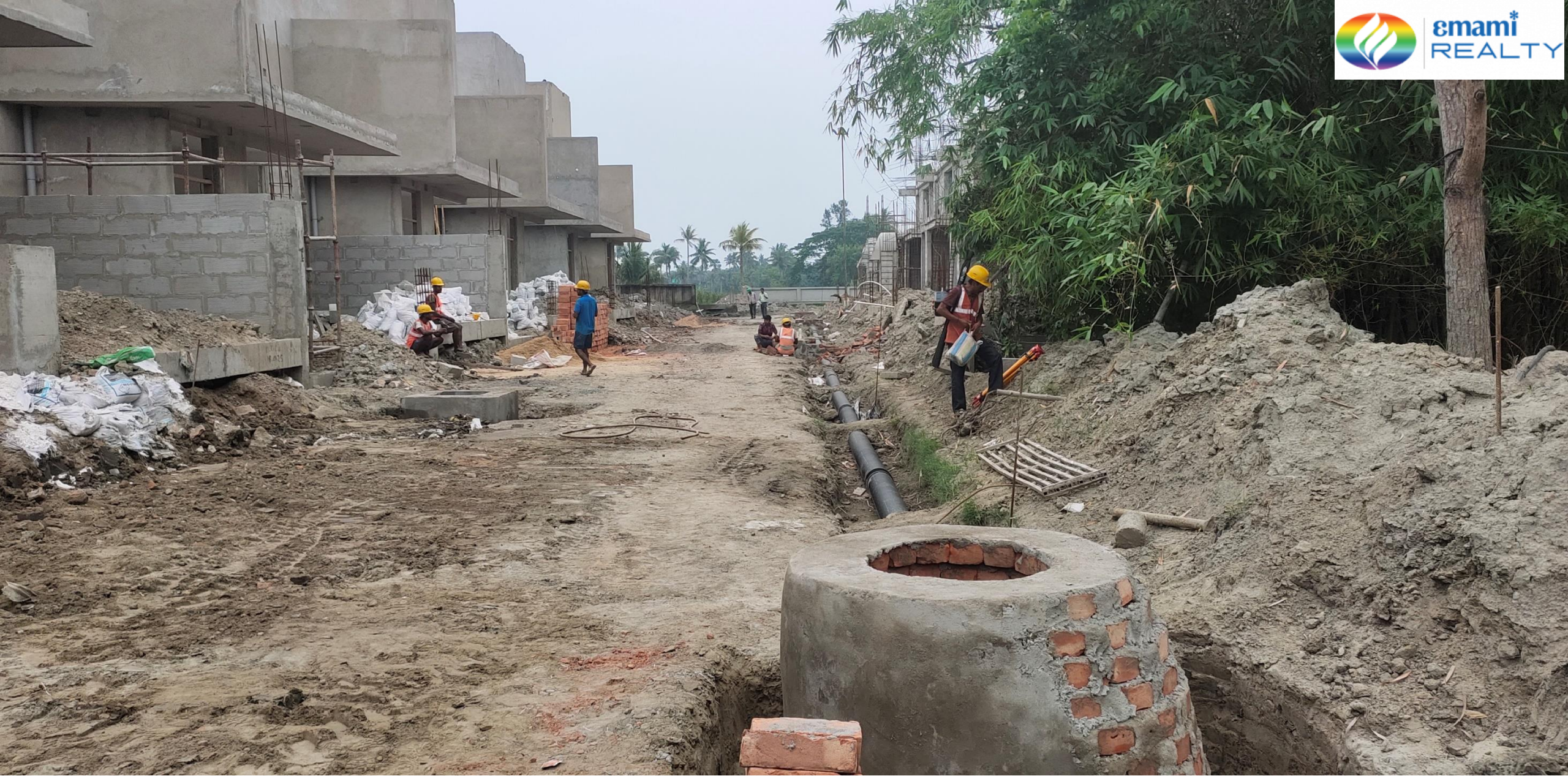
PROGRESS PHOTOGRAPHS: SERVICES WORK IN INTERNAL ROAD
